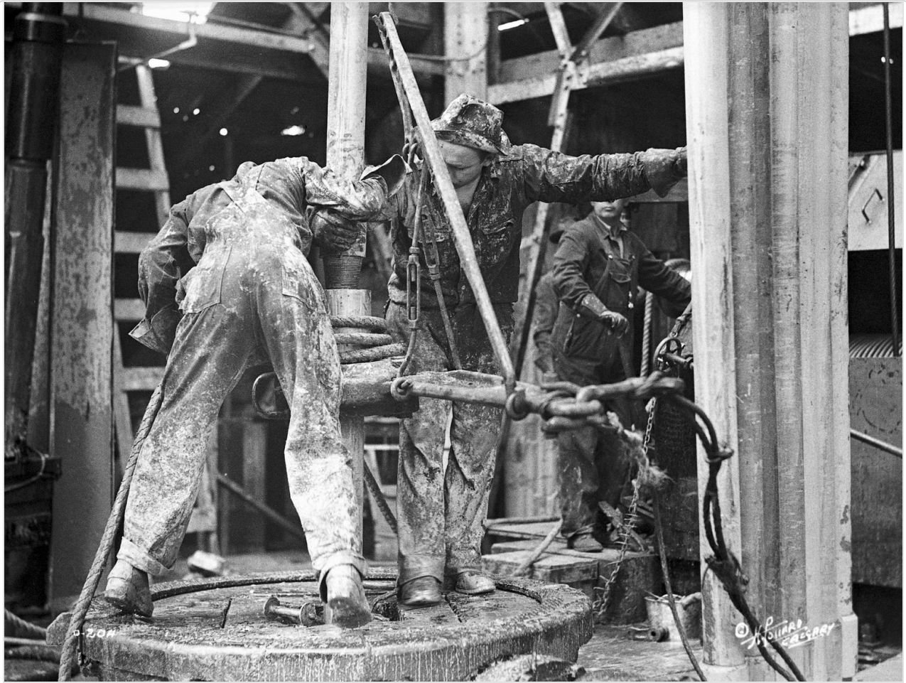
On the drilling floor in the Turner Valley field, where the province's oil began. Photo: Provincial Archives of Alberta (no known copyright restrictions), via Wikimedia Commons.
