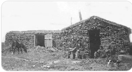
A prairie sod house — the kind of first home a homesteader like Ernest built by hand.
